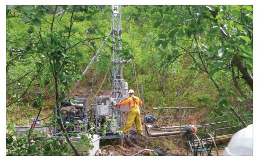
Left, contractor crews performing boring tests to help determine the geological conditions of the project
