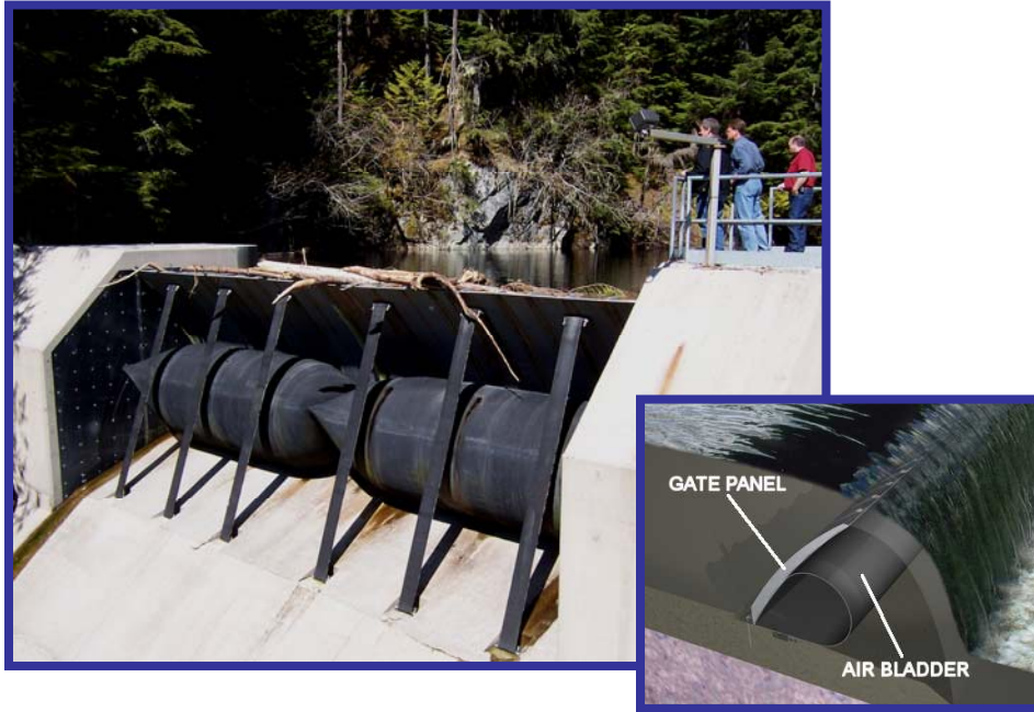
Figure 1.4 Typical Obermeyer Gate Installation
