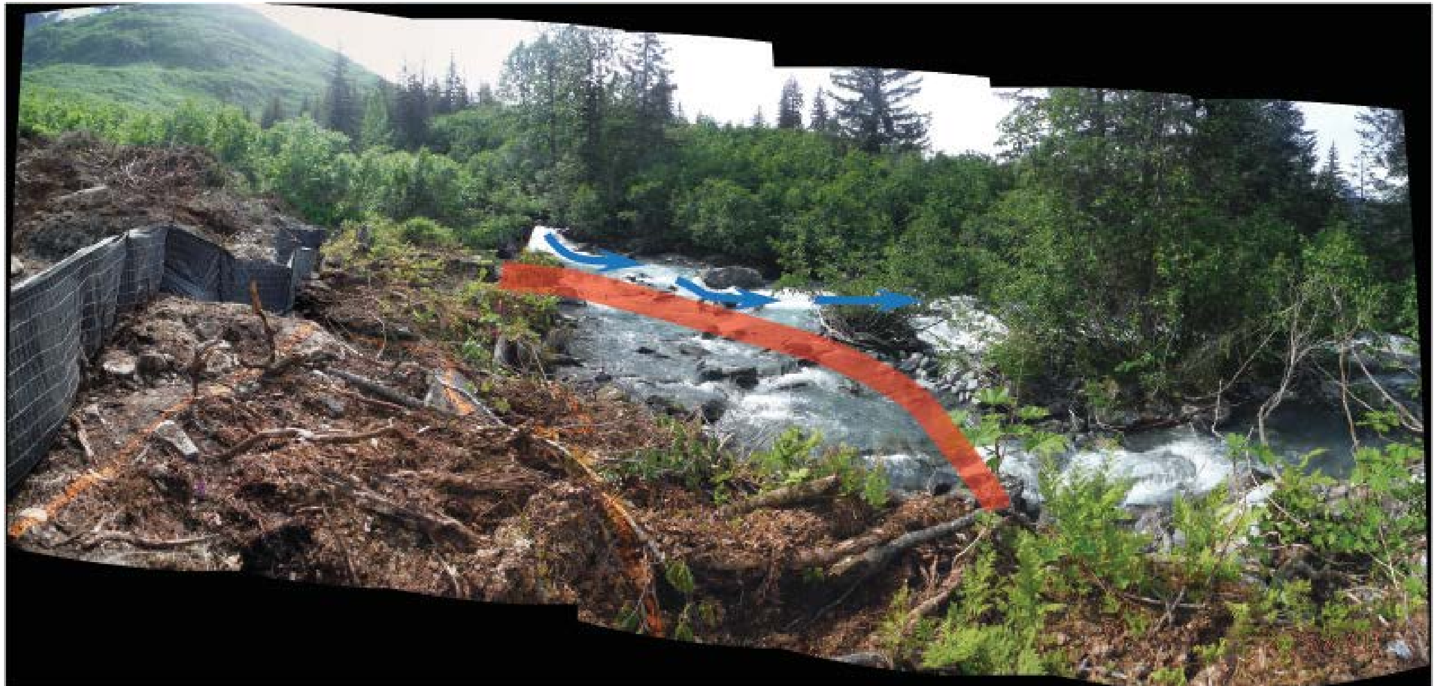
Figure 2. Photo taken 6/20/2014 looking upstream at the tailrace location.
