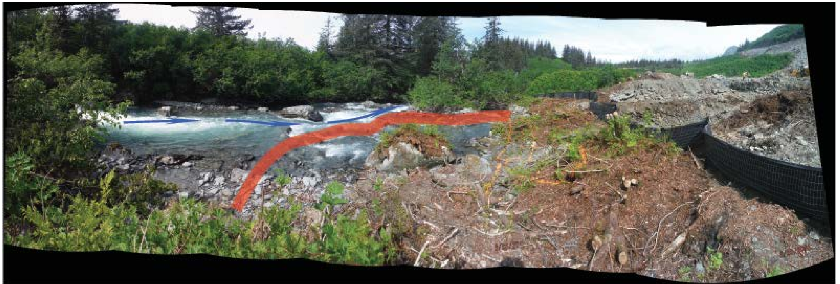
Figure 3. Photo taken 6/20/2014 looking downstream at the tailrace location.
